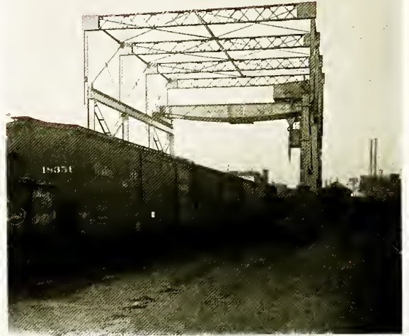
C. R. R. of N. J. Electric Crane, for Handling Heavy Freight
